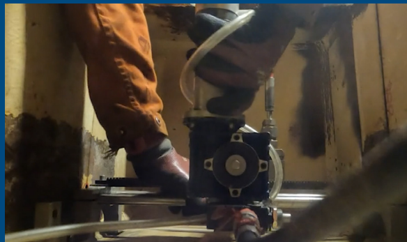
UHP Cutting Tool Offshore in Use
